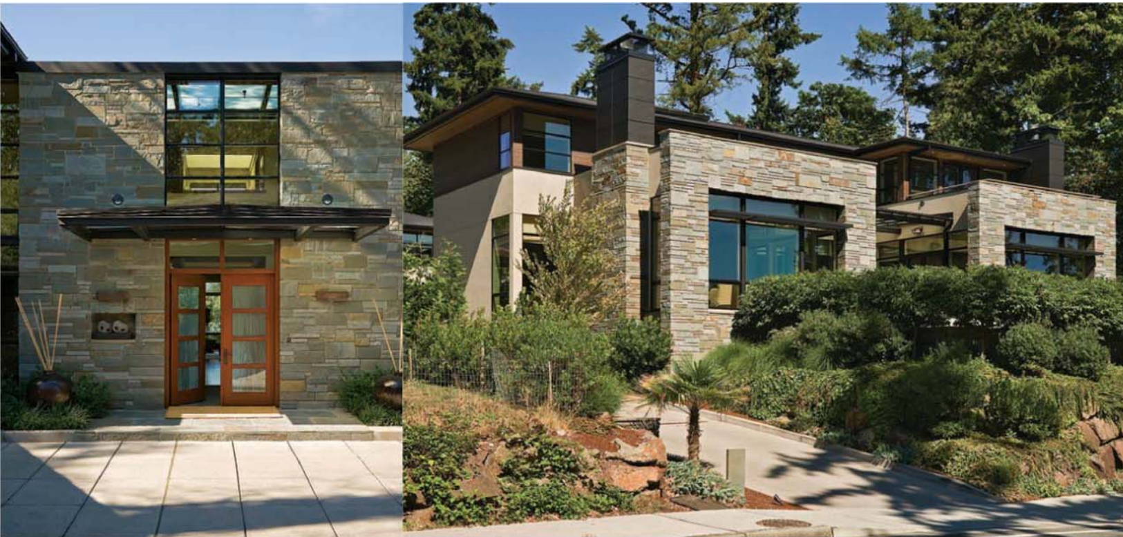
OPPOSITE: ARTECH FINE ART SERVICES INSTALLED MUCH OF THE ARTWORK AND ANTIQUES, INCLUDING THE PALM LEAF BRONZE WHEELS BY SINGAPOREAN ARTIST CHRISTOPHER NOTO. ABOVE: THE EXTERIOR OF THE HOME IS COVERED IN ASHLER-PATTERNED PENNSYLVANIA BLUESTONE.
